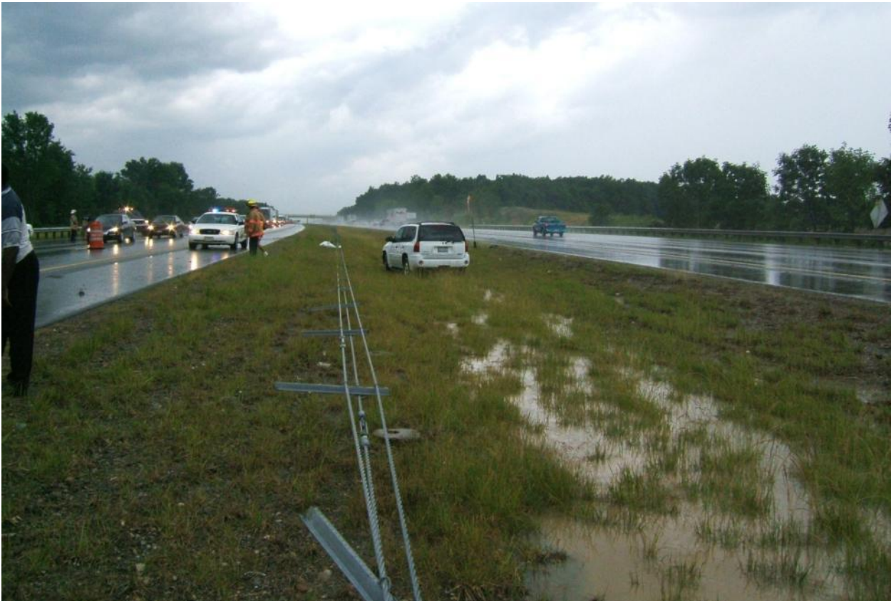
Figure 48. Override Penetration Crash Caused by Strong Cable-to-Post Attachment
