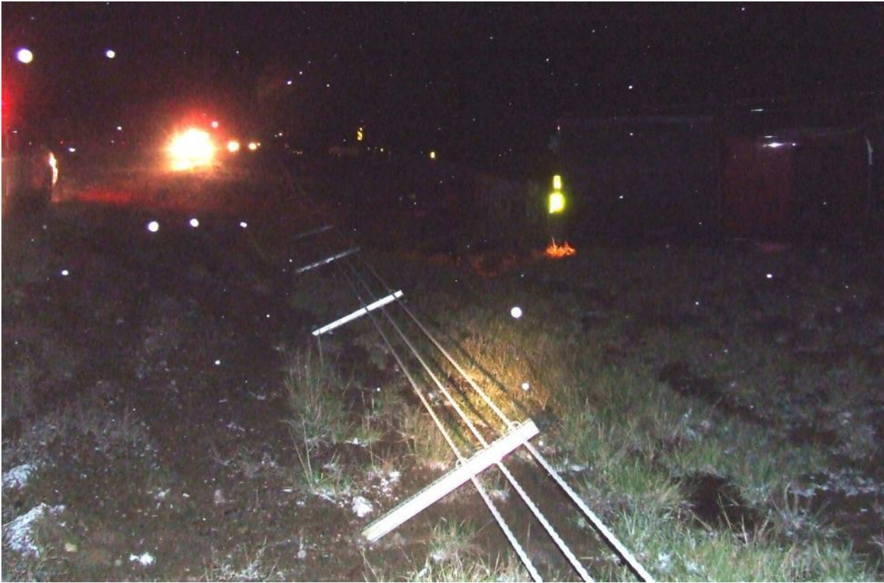
Figure 46. Penetration Crash Caused by Strong Cable-to-Post Attachment
