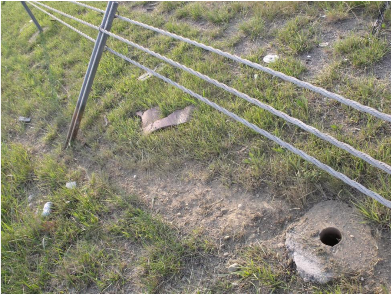
Figure 50. Prying Penetration Crash on Nucor NU-CABLE Barrier
